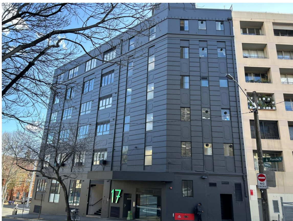
Figure 5 – View of Randle Street Frontage of Existing Building – 17 Randle Street (Source: City of Sydney)
